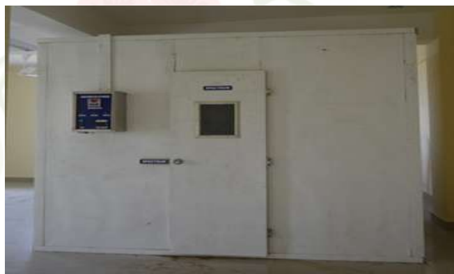
Fig 74. Installation of model cold storage unit of 15000 liters capacity
